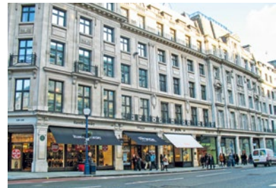
Kingsland/Carrington House, W1
