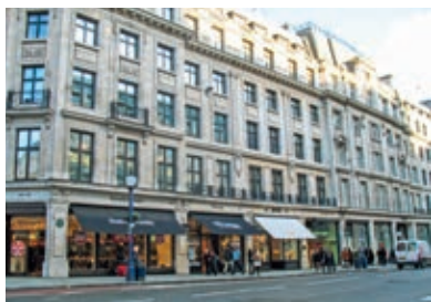
Kingsland/Carrington House, W1
