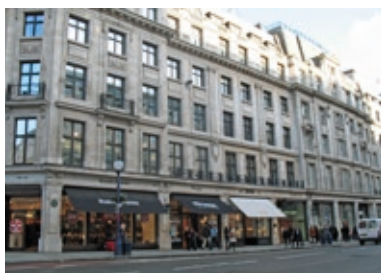
Kingsland/Carrington House, W1
