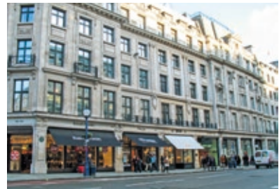
Kingsland/Carrington House, W1
